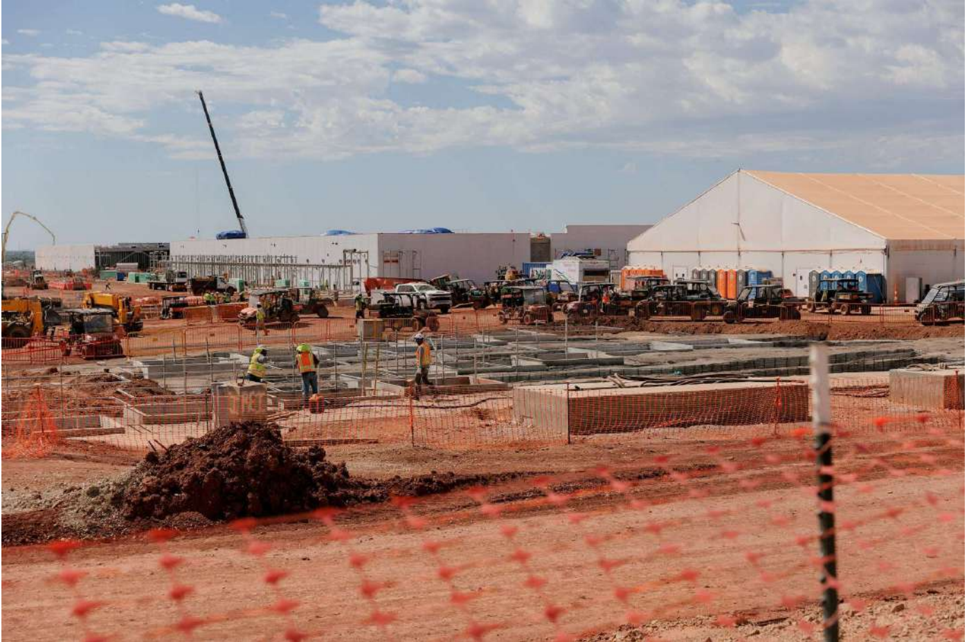
Data center buildings are under construction in Abilene, Texas, U.S., September 23, 2025. REUTERS/Shelby Tauber/Pool/File
